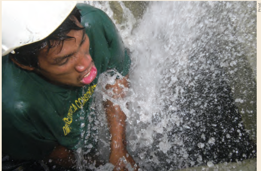
Full commitment at the pipe burst repair
